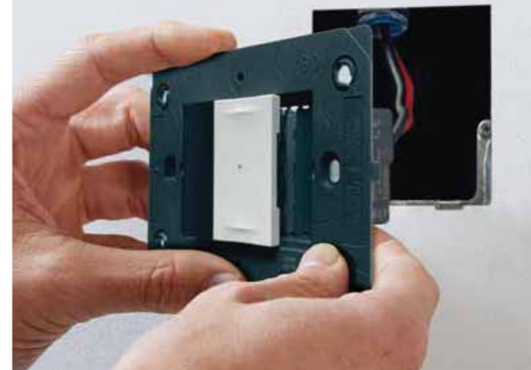
INSTALL NEW SMART DIMMER SWITCH ON WALL
